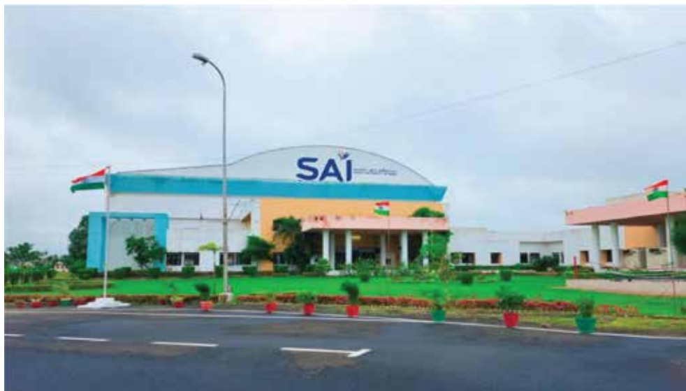
Udhav Das Mehta (Bhai ji) Central Centre, Bhopal
