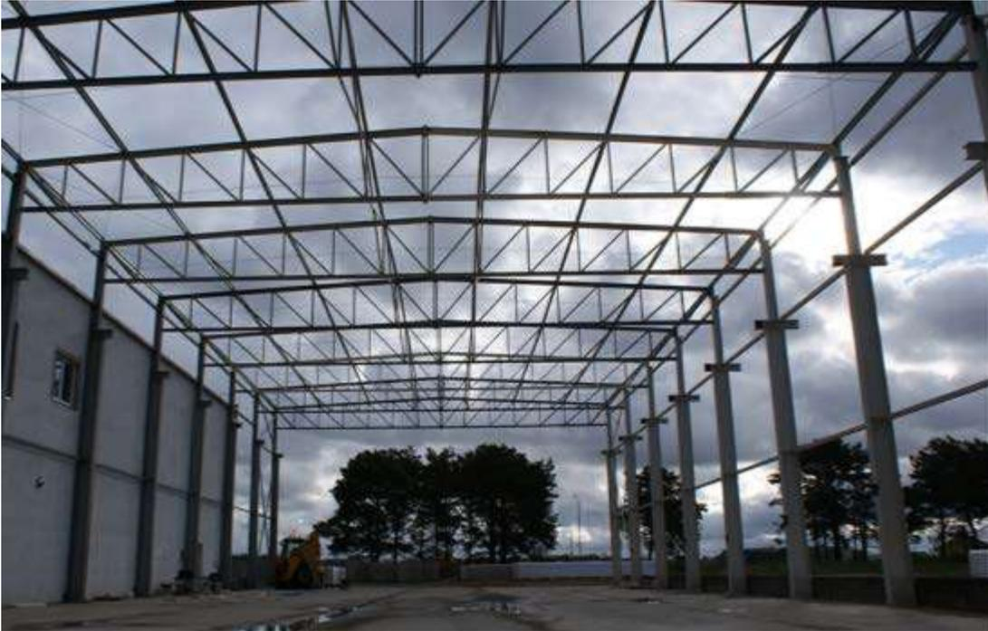
COMBINATION OF STEEL & RCC STRUCTURE
